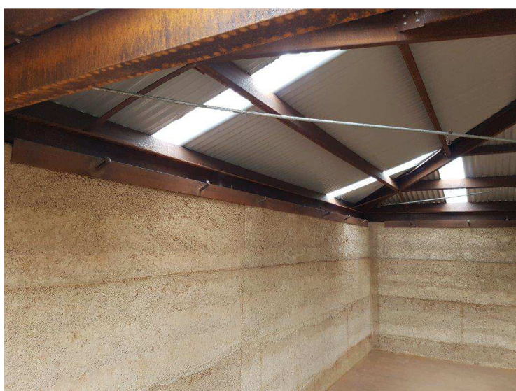
Trial of hooks at rammed earth shelter using recycled materials
