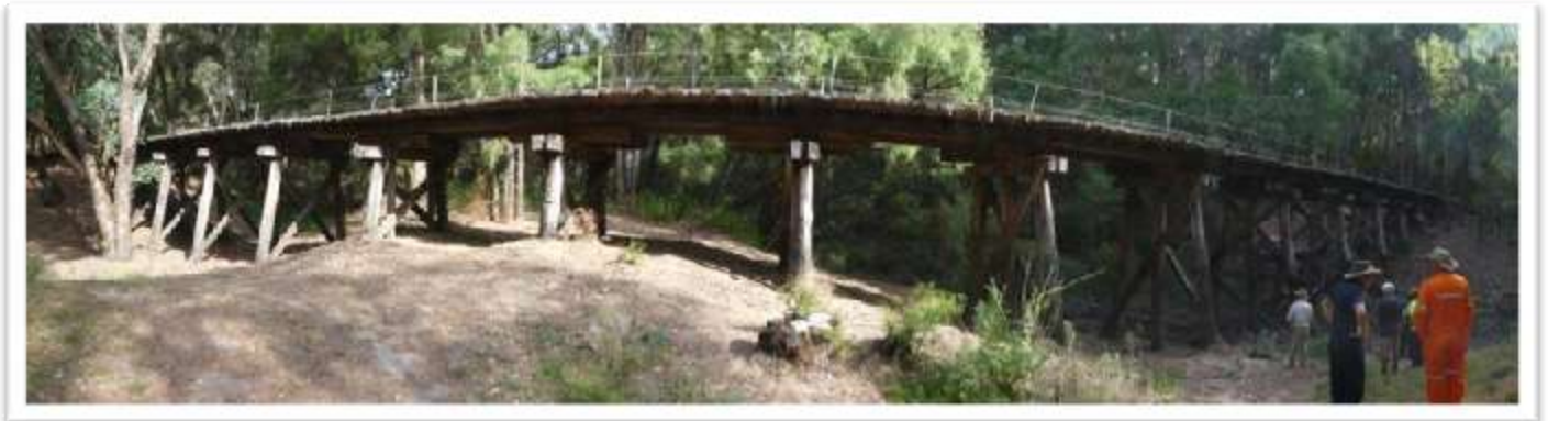
River Road Bridge near Pemberton
