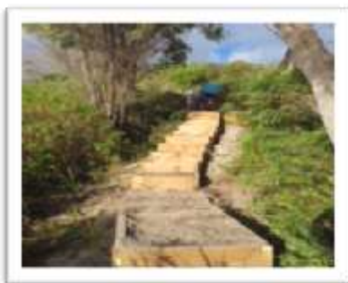
Steps installed up the dunes at Irwin Inlet.
