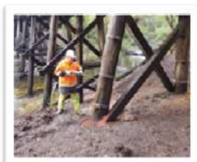
Preservation work on River Road Bridge.
